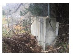
There is also a manhole on the slope behind the building (MH-01) on the outfall pipe that appears to be leaning significantly downhill that should be repaired.
