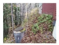
protection. The wing retaining walls have suffered from freeze thaw damage where the steel fence posts were cast in place. This will need repair to ensure fence stability.
