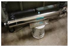
disinfection units, one of which is non-functional. The original Basis of Design specified units rated for 15 gpm, though subsequent upgrades increased the unit sizes to 40 gpm. A hypochlorite system is currently provided for a backup. The functional UV unit was installed in 2018.
