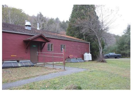
last replaced in 2008, has leaked as evidenced by water damage visible in the laboratory/office space. Exterior paint is peeling, and doors are rusting. The exterior garage door is inoperable.
