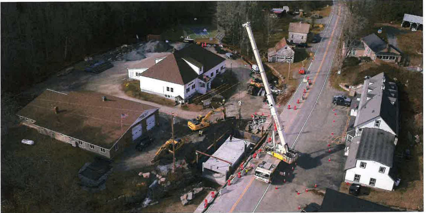
Installation of the new culvert at the Municipal Center on November 10, 2025. Drone photo by James Weber.
