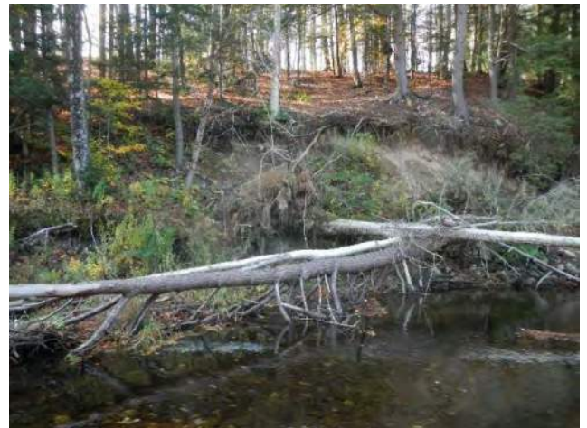
Figure 4.15: Mass failure on reach M05.
