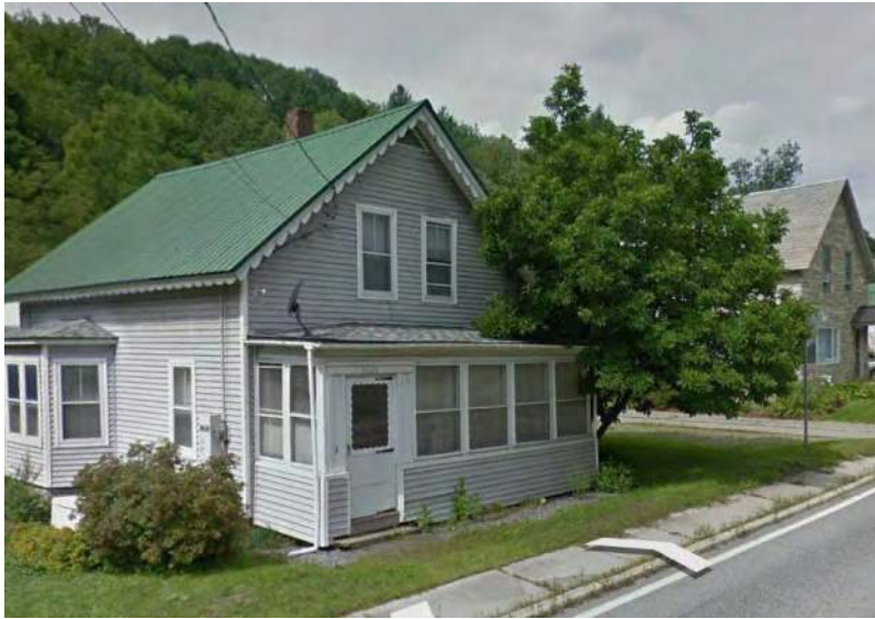
VT Route 100, view northwest
