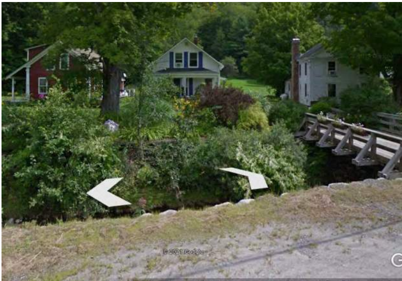
VT 112, view northeast
