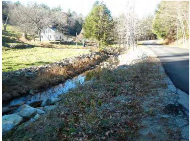
Figure 4.18: Bank armoring, encroachment, and straightening on reach T1.02.
