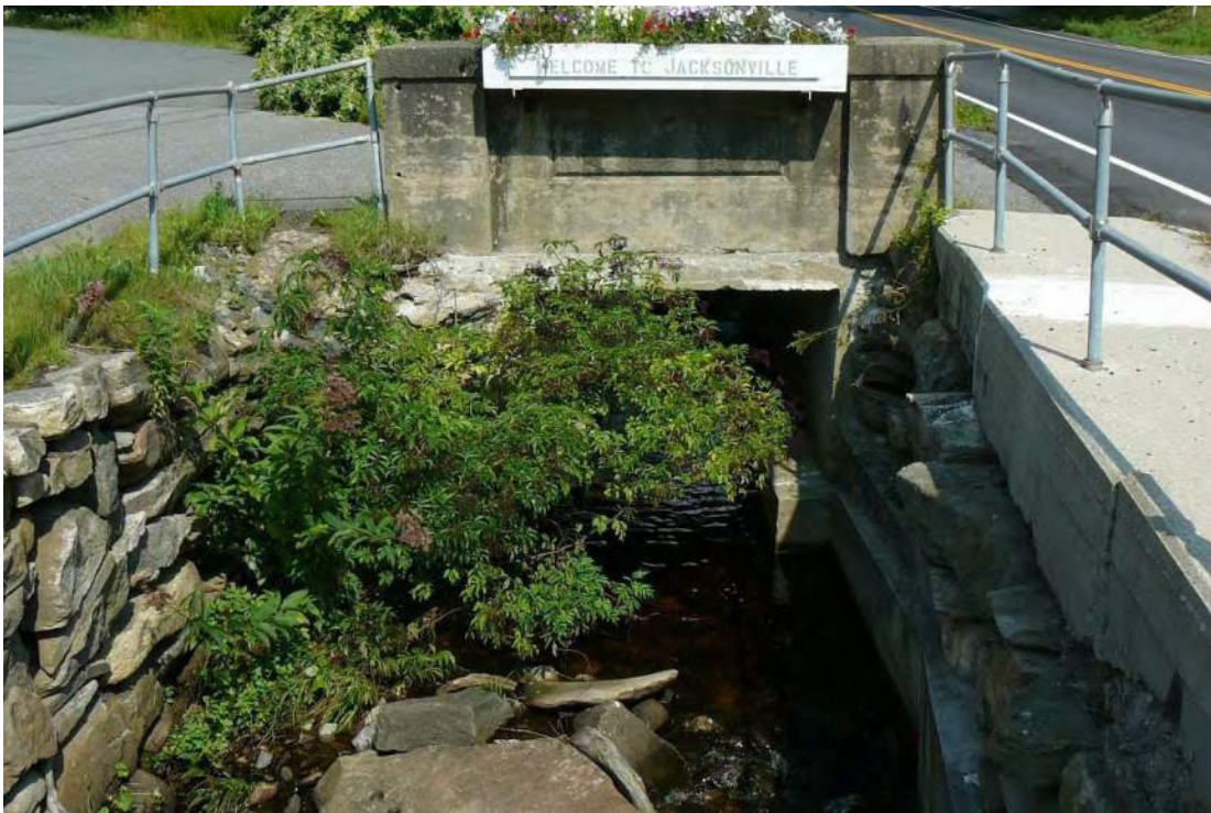
Figure 30. View northwest of downstream rail of concrete bridge.
