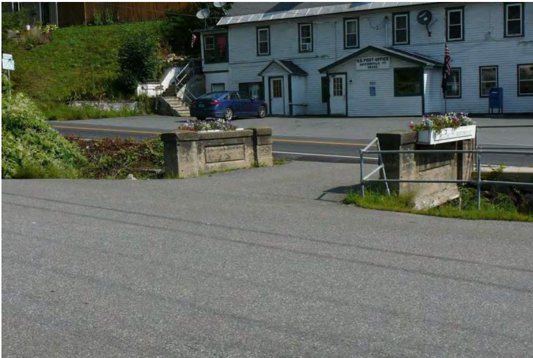
Figure 26. View northeast of concrete bridge.
