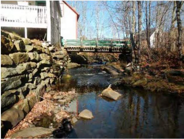
Figure 4.10: Extreme bank armoring on reach M06.B.
