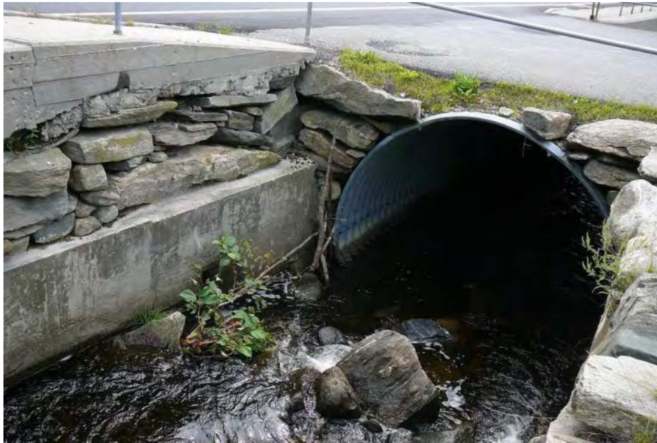
Figure 32. View southeast of inlet/upstream end of culvert.
