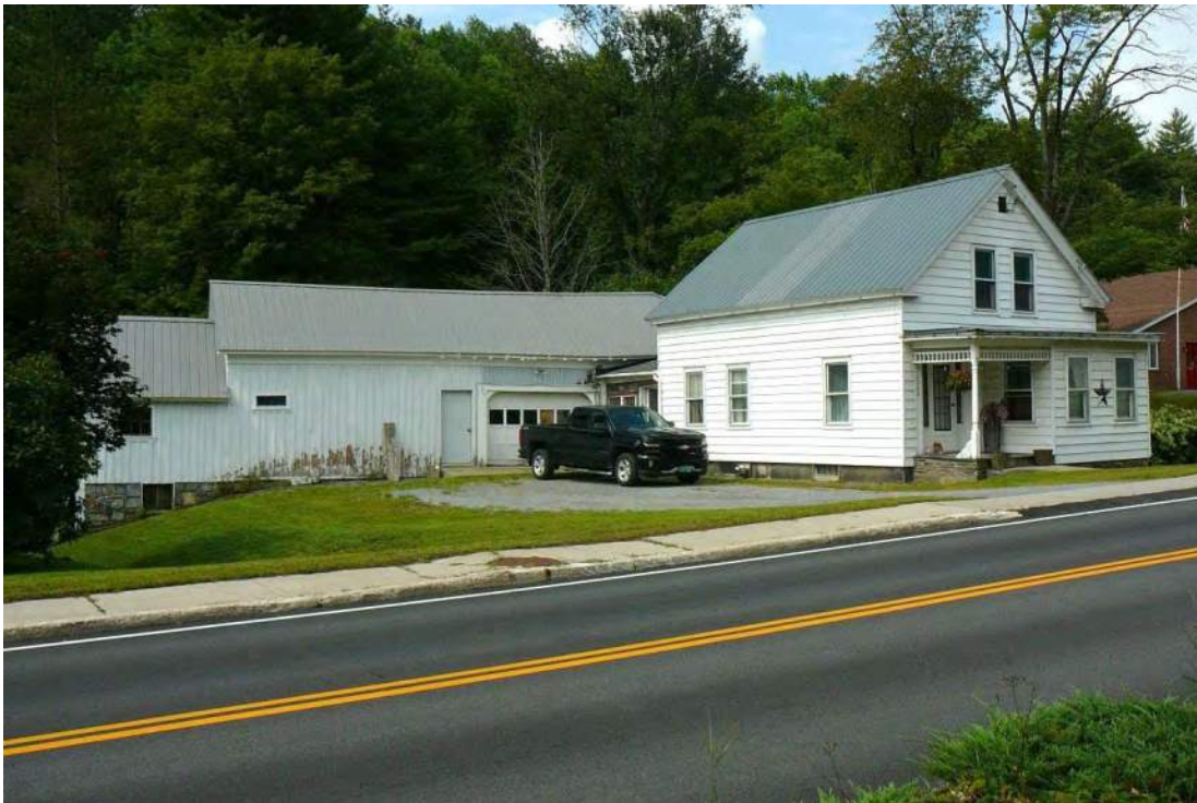
Figure 36. View northwest of the house at 2984 VT Route 100.
