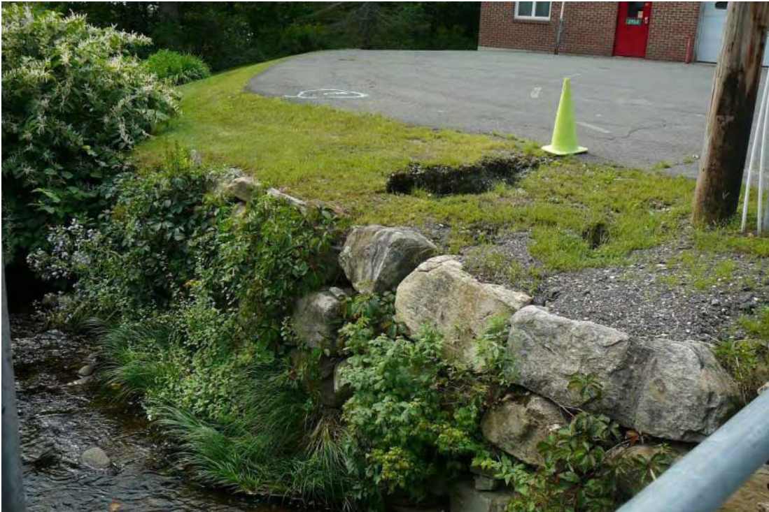
Figure 19. View southwest of the project area showing fill, utility pole and paving in front of the Fire House.
