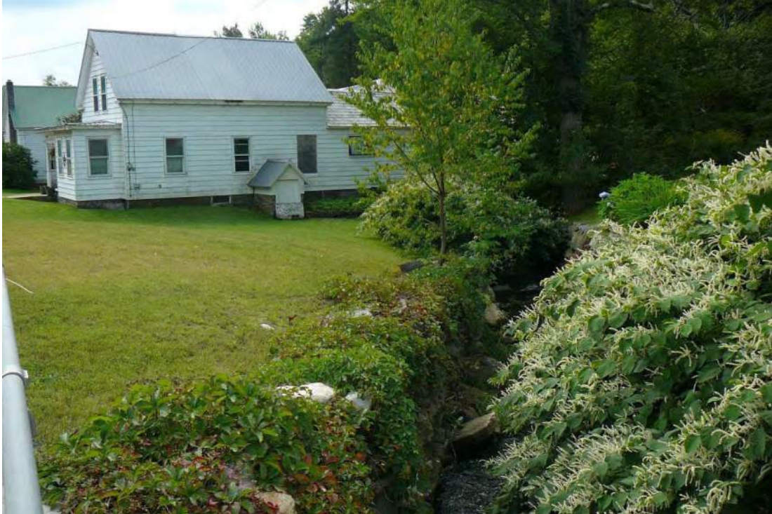
Figure 20. View southwest of the project area showing area of fill to the north of house at 2984 VT Route 100.
