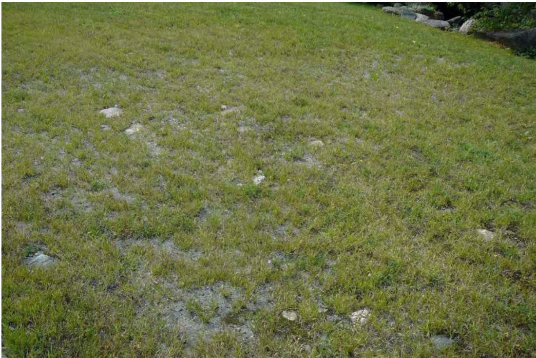
Figure 21. Close-up view southwest of fill to the north of house at 2984 VT Route 100.
