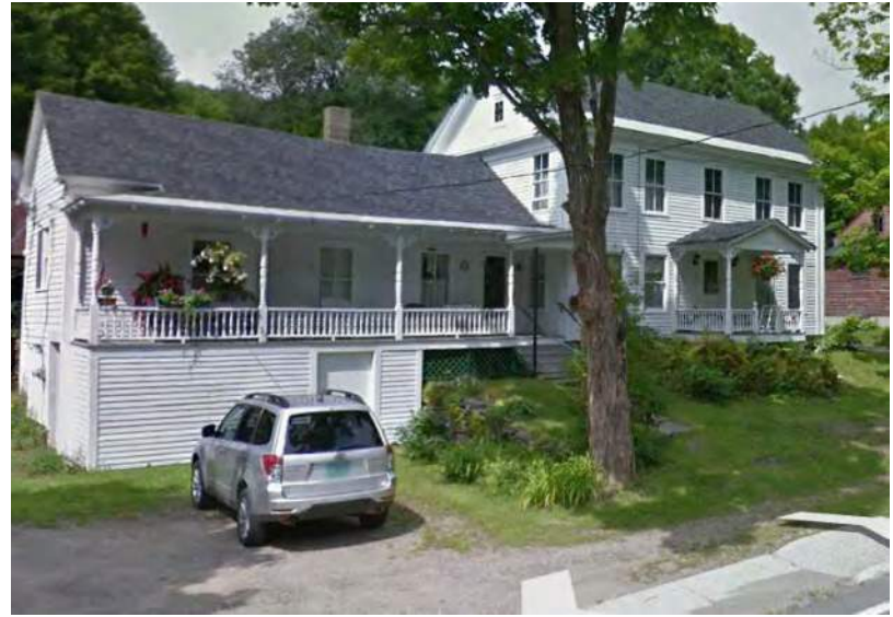
VT 112, view northwest
