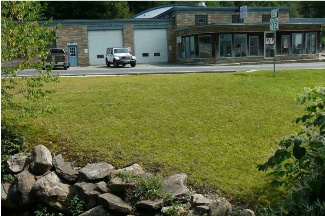
Figure 6. View east of the project area across VT Route 100 from in front of the fire department; stone-lined bank of East Branch North River in foreground.
