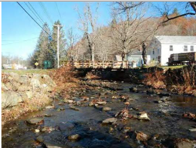
F-type channel due to straightening and armoring.
