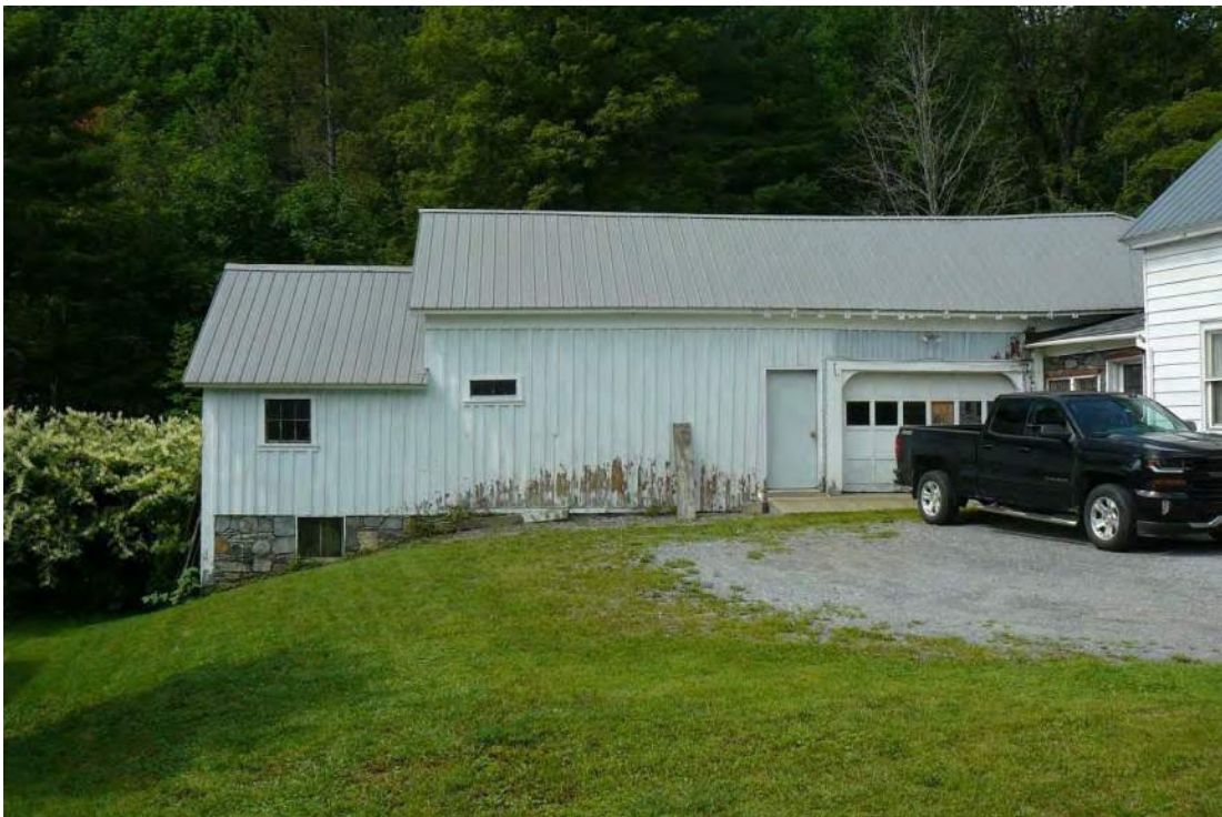
Figure 23. View west of the project area showing area of probable fill/land disturbance to the east of house at 2984 VT Route 100.
