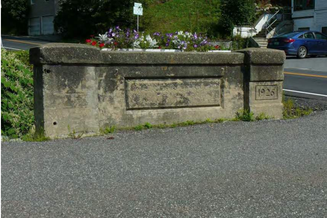
Figure 28. View northeast of upstream rail of concrete bridge.
