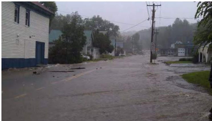
Figure 5.1: Tropical Storm Irene floodwaters overtopping the culvert and bridge at the Whitingham Municipal Center and flowing south down VT 100 (photo courtesy of G. Havreduk).
