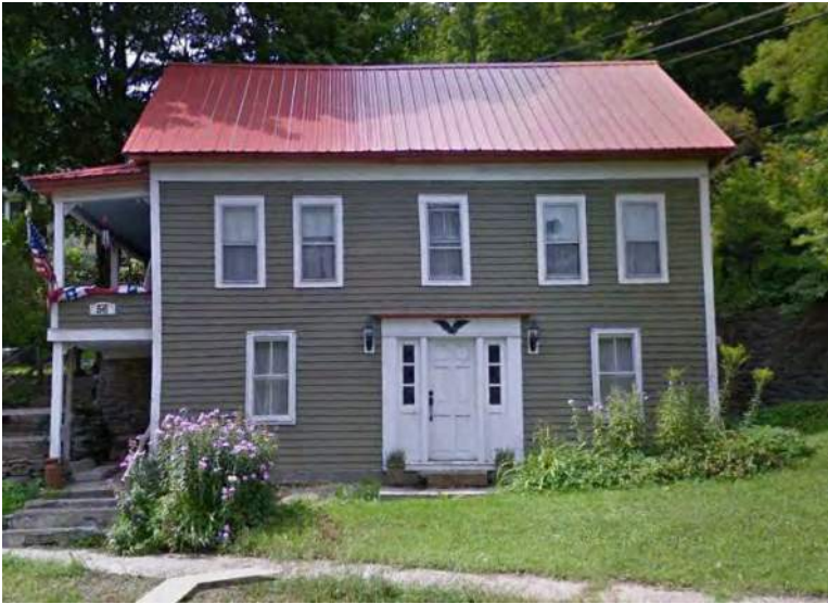
VT 112, view southwest
