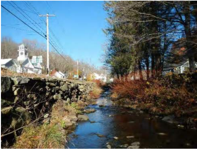
Figure 4.17: Extreme straightening along segment M06.B.
