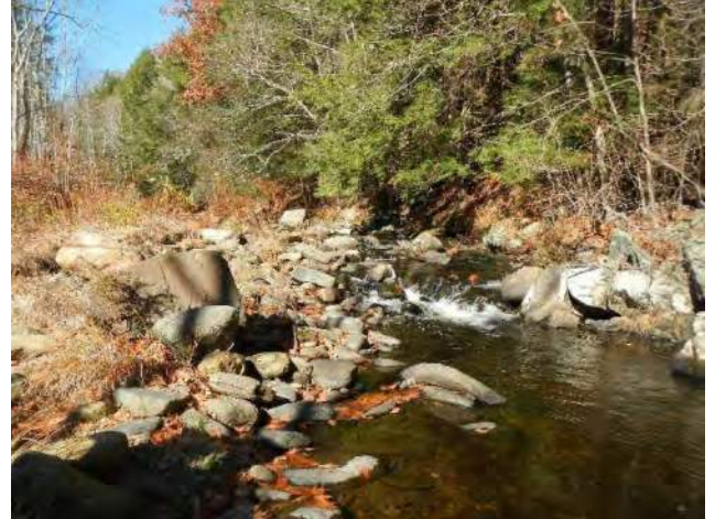
Figure 4.7: Grade controls in reach M05.
