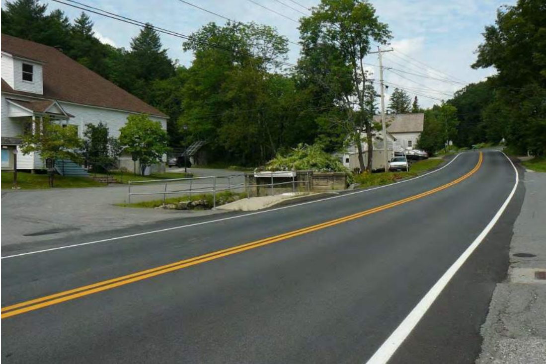
Figure 18. View northwest of the project area showing structures and paving in front of the Municipal Center.
