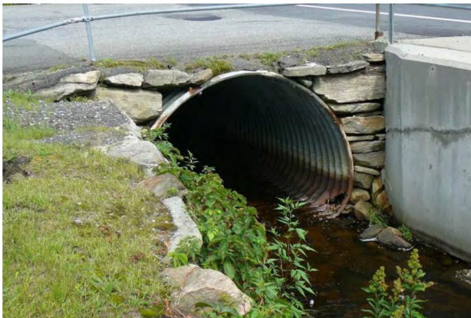
Figure 33. View northeast of outlet/downstream end of culvert.
