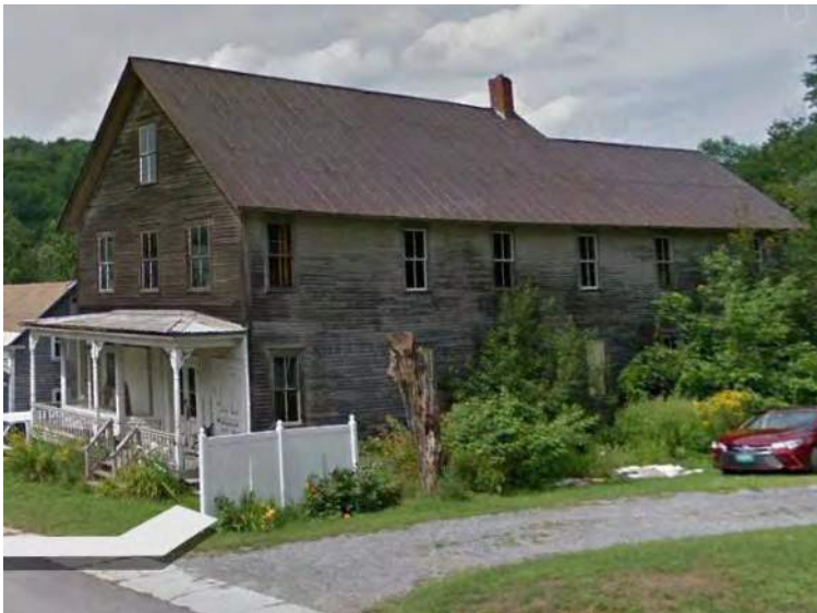
Gates Pond Road, view west
