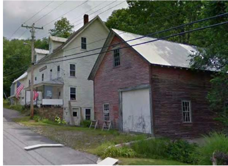
Gates Pond Road, view northeast
