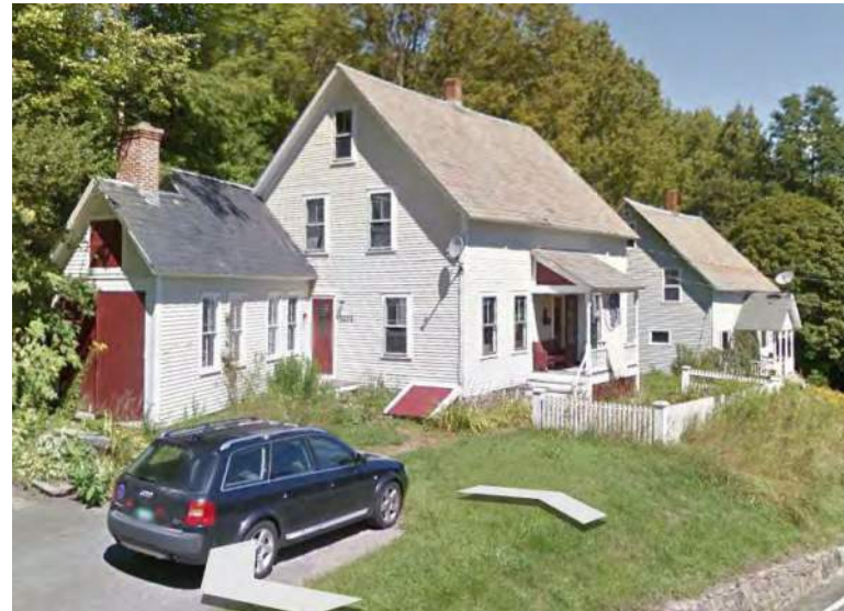
VT Route 100, view north
