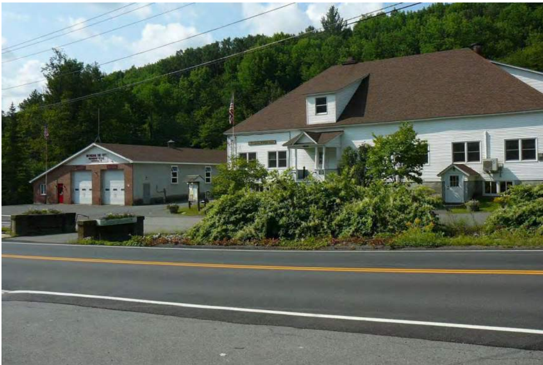
Figure 4. View southwest of the project area along VT Route 100; fire department building at left, municipal building at right, 1926 bridge at left foreground.
