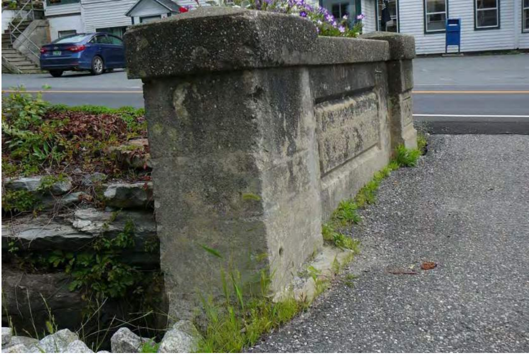
Figure 29. View northeast of upstream rail of concrete bridge.
