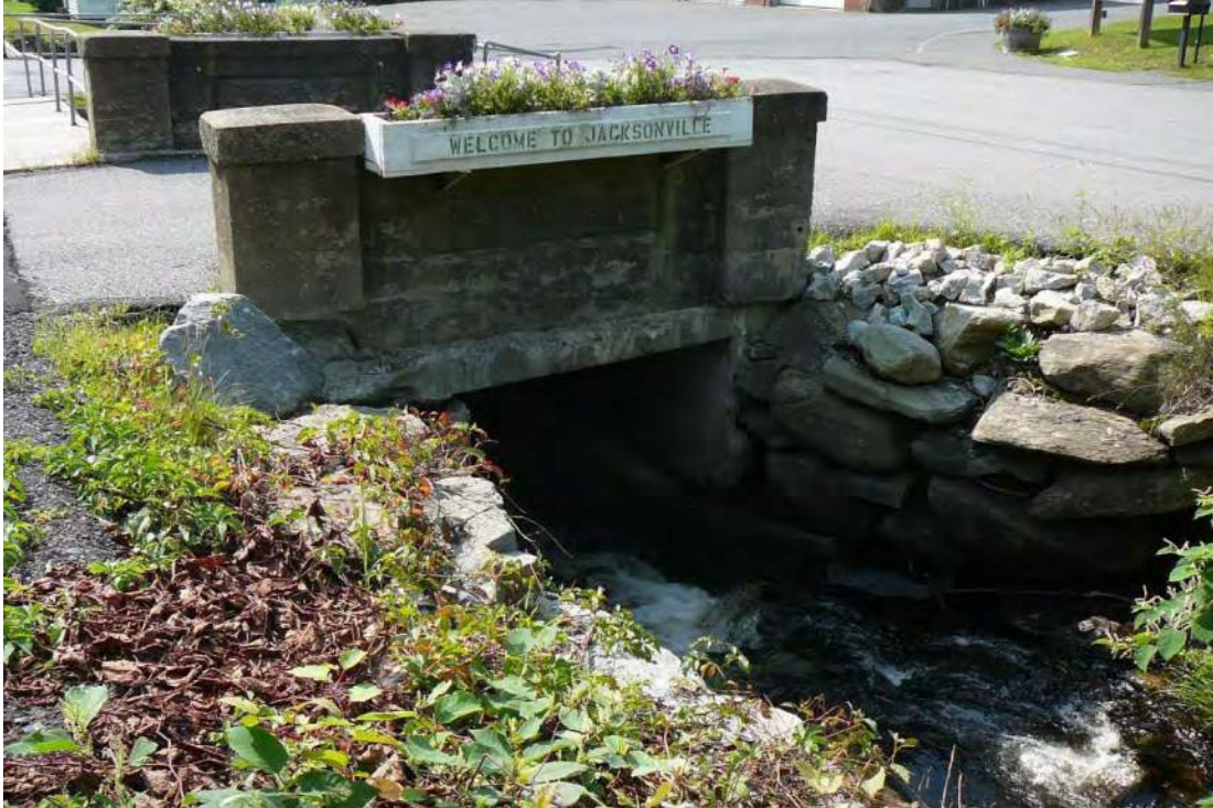
Figure 27. View northeast of concrete bridge.
