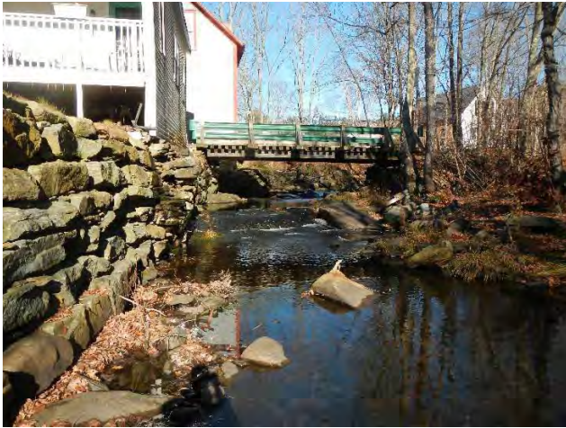
Figure 4.10: Extreme bank armoring on reach M06.B.
