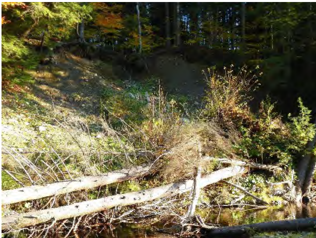
Figure 4.14: Mass failure on segment M03.C.
