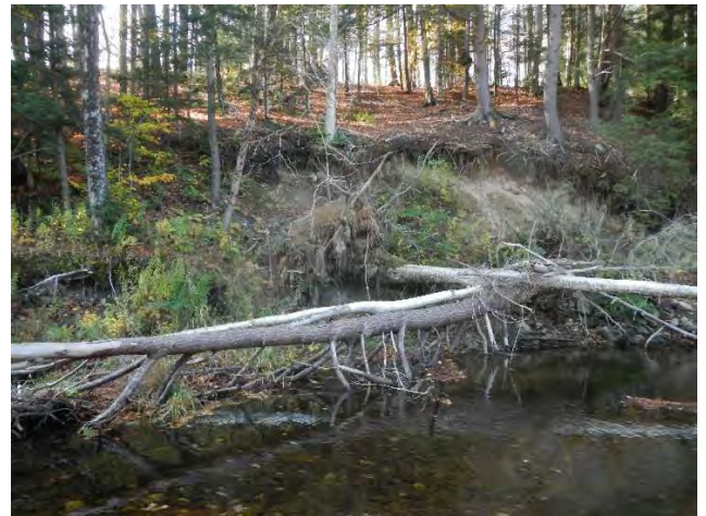
Figure 4.15: Mass failure on reach M05.
