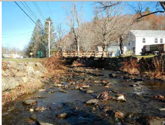
F-type channel due to straightening and armoring.
