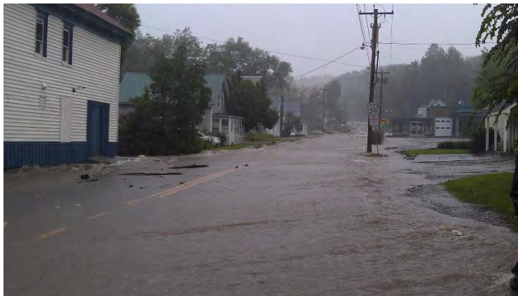
Figure 5.1: Tropical Storm Irene floodwaters overtopping the culvert and bridge at the Whitingham Municipal Center and flowing south down VT 100 (photo courtesy of G. Havreduk).
