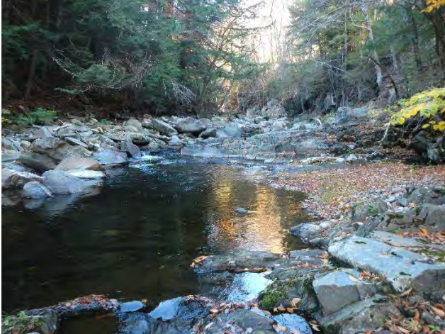
Figure 4.6: Grade controls in segment M03.B.
