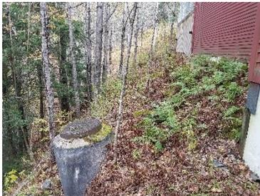
There is also a manhole on the slope behind the building (MH-01) on the outfall pipe that appears to be leaning significantly downhill that should be repaired.
