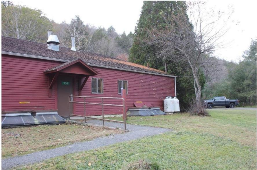
The building is exhibiting signs of its age in many of the building subsystems. The roof, last replaced in 2008, has leaked as evidenced by water damage visible in the laboratory/office space. Exterior paint is peeling, and doors are rusting. The exterior garage door is inoperable.
