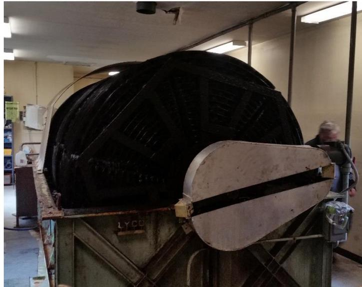
The clarifier tank is in fair condition with most of the paint and interior bituminous coating intact. These tanks remain serviceable but would benefit from new interior and exterior coatings to extend their useful life.
