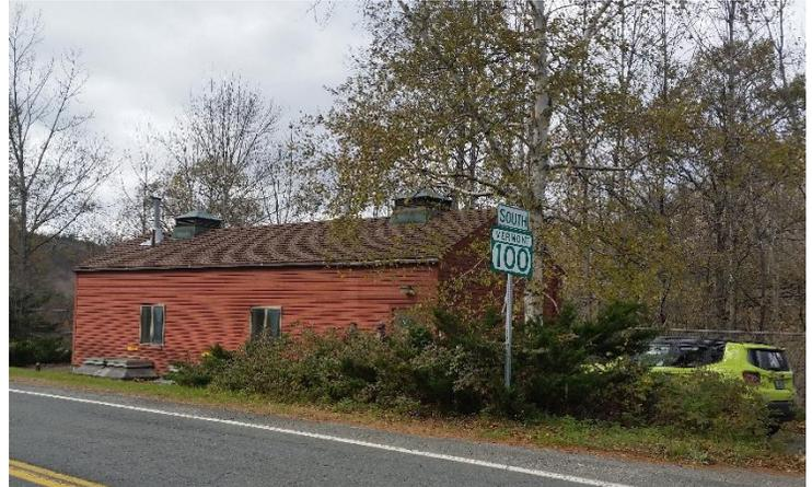
Overall the building is generally serviceable but is in need of improvements to doors, interior and exterior wall surfaces and building electrical, lighting and HVAC systems are old and their condition, function and reliability are marginal and warrant rehabilitation or replacement for continued reliable long term occupancy.
